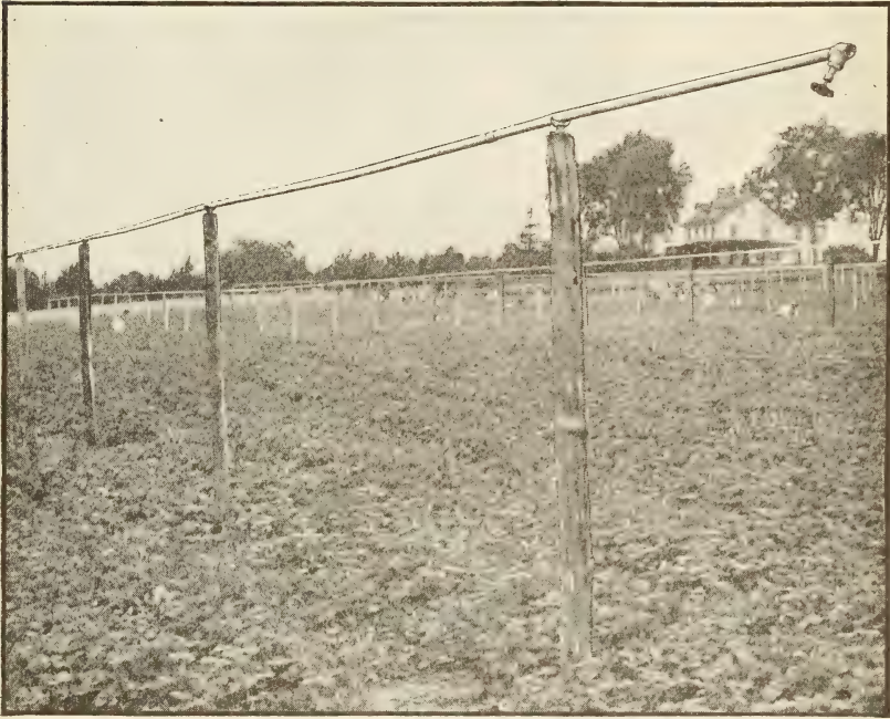
FIG. 13.—Overhead spray nozzle lines mounted on wooden posts 6½ feet above the ground. [Farm of Granville W. Leeds, Rancocas, N. J.]
